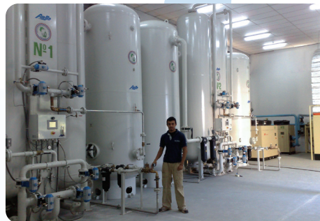
AS-Z5500-HM Duplex PSA Medical Oxygen Plant — Paraguay
