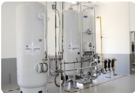
AS-Q2600-HM Duplex PSA Medical Oxygen Plant — Nicaragua
