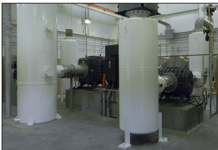
Silencers for vacuum blower discharge (left front), feed air intake (right front), vacuum blower suction inlet (left rear), and feed air blower discharge (right rear) complement user-friendly operator interface.
