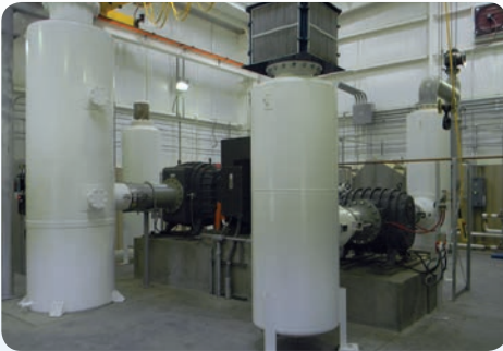
Inlet and Discharge Silencers
