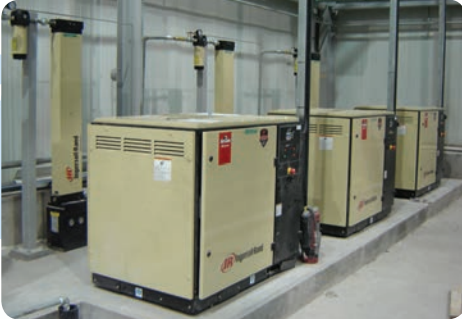
Instrument Air Compressor
