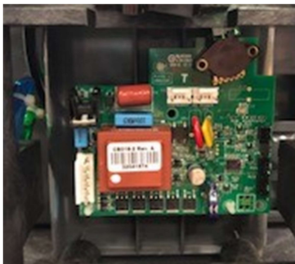
Figure 14. Board reinstalled onto superstructure.
