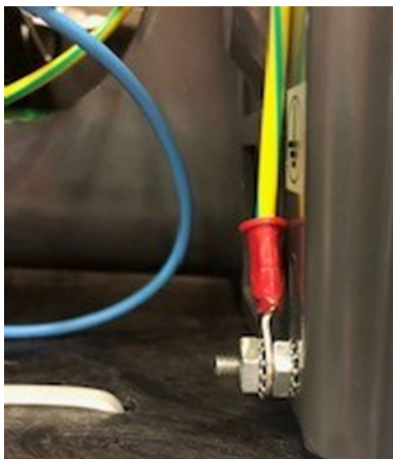
Figure 76. Showing ground wire and nut re installed.
