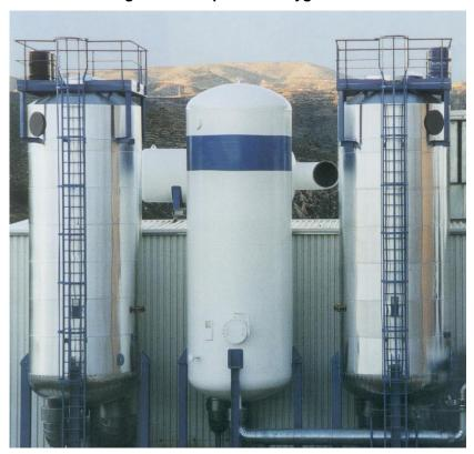
Figure 4 Example of an oxygen VSA
