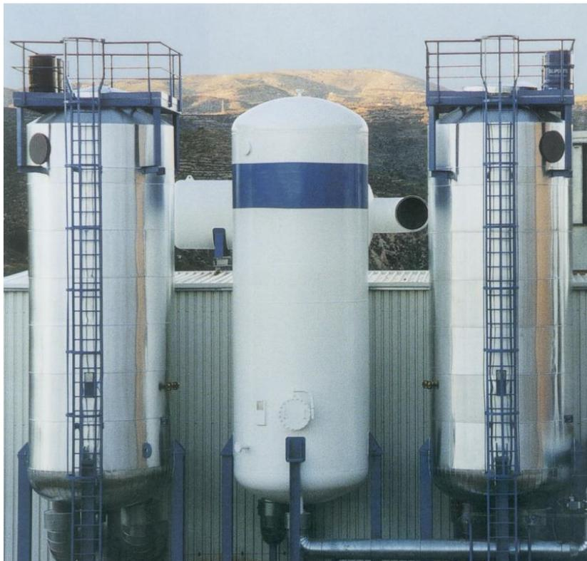
**Figure 4 Example of an oxygen VSA**
