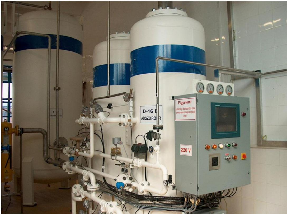
Figure 9 Example of a nitrogen generator
