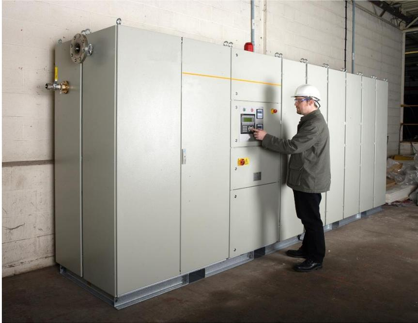
Figure 12 Example of a nitrogen membrane
