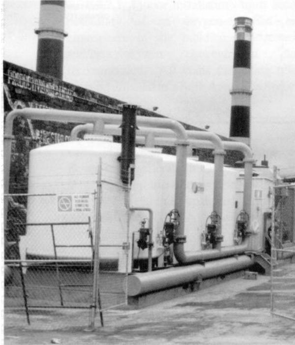
**Figure 5 Example of a three bed oxygen PSA**
