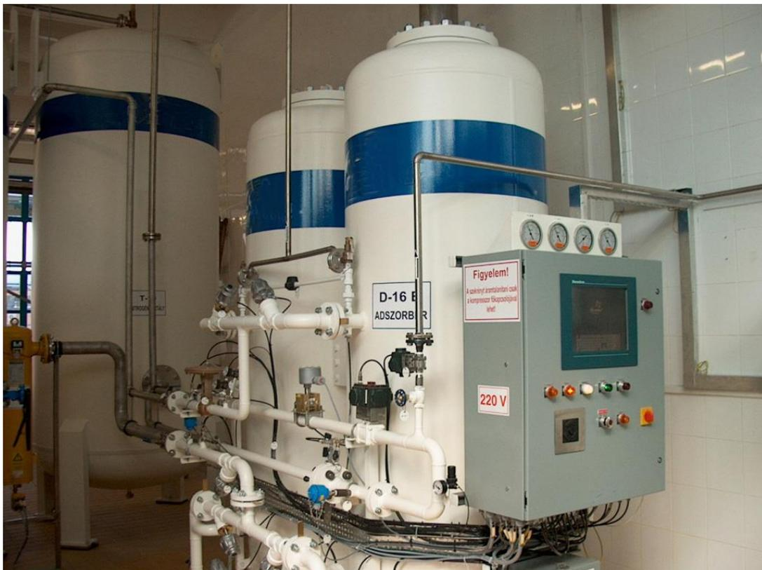
Figure 9 Example of a nitrogen generator
