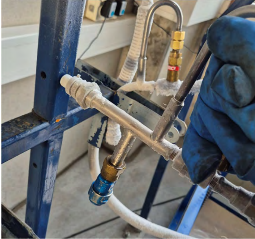
Figure 5 – purging transfer hose.
