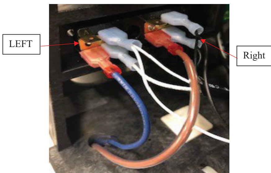
Figure 19. 120V terminal block connections.
