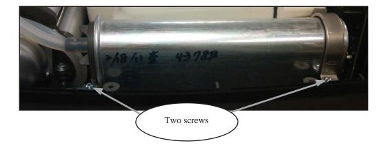
Figure 37: Remove Screws
