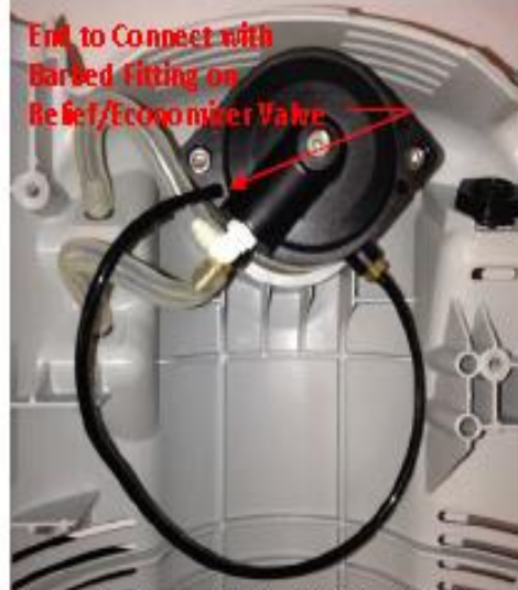
Figure 6. Current Style HELIOS with Plug and Nut (Some components removed for clarity).
